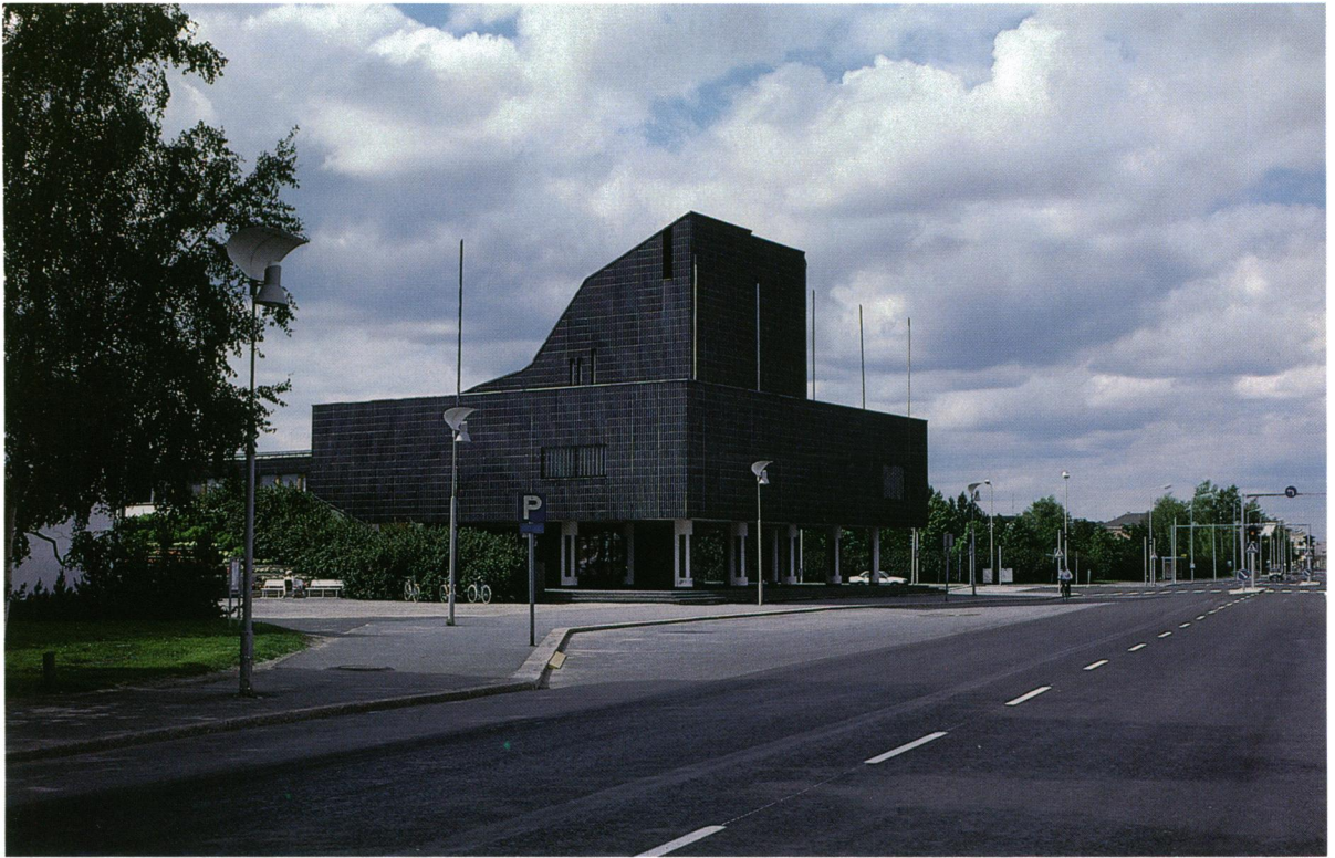
Fig. 17. Entry and council chamber, Town Hall, Seinäjoki, Finland, 1963–65. Photograph by the author.
